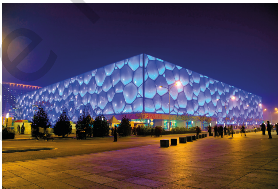
FIGURE 15.4.1 The outer shell of the Water Cube Stadium in Beijing, China, is made of ETFE, a new copolymer building material.
